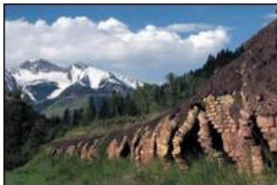
The historic coke ovens in Redstone, clearly visible from Highway 133, were preserved through partnerships with several organizations in 2004. (ED KOSMICKI)
